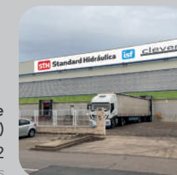
Getafe (Madrid, ES) Superficie 6.500 m2 Facilities / Installations
